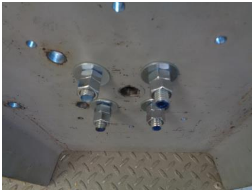
Photo No. 10 Post Mount Connection Simulated Concrete Bolted Through Bottom Spacer (Bottom Side)
