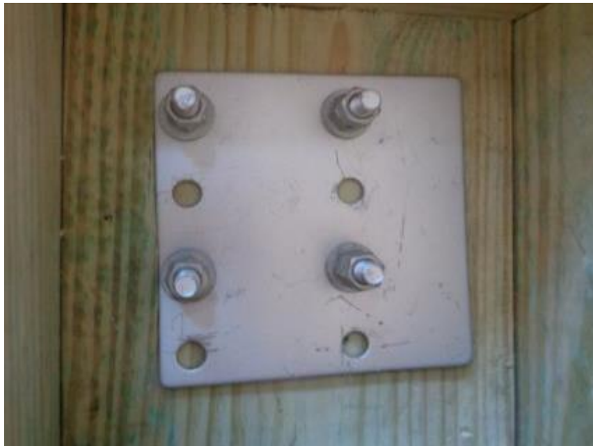
Photo No. 6 Post Mount Connection Mock Wood Deck (Bottom Side)
